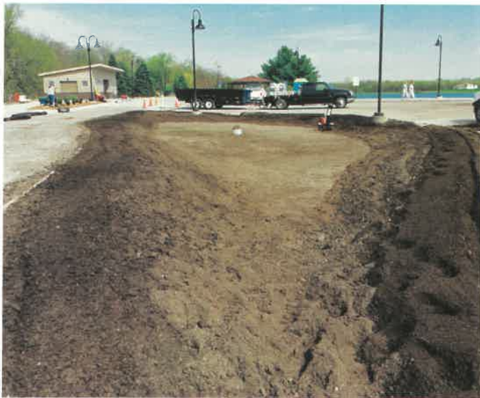
STEP 3 Placing the Soil Media
