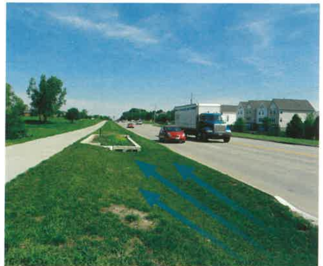
Pre-treatment swale for Ankeny biocell
