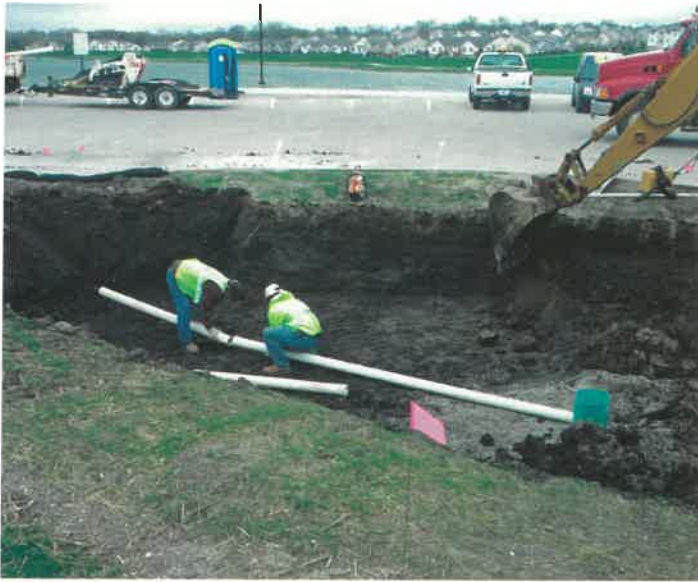
STEP 1 Excavation and Installation of the Subdrain
