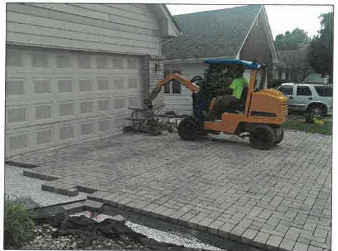
Step 4 Laying pavers
