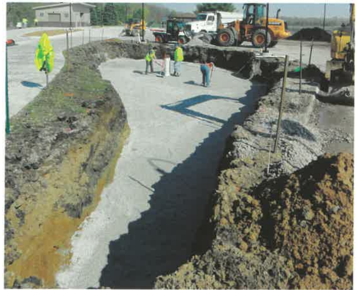
STEP 2 Installation of Rock and Overflow Pipe
