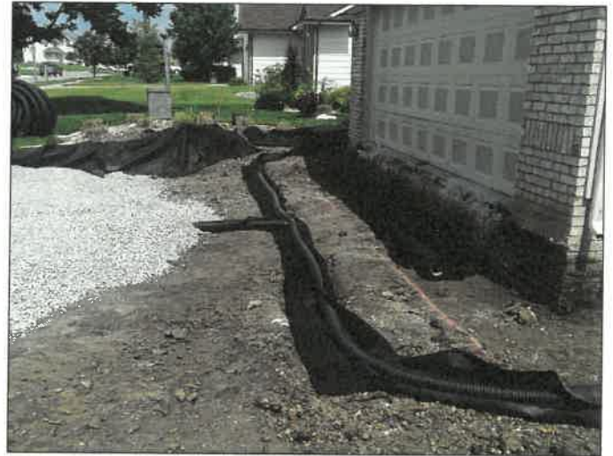
Step 2 Installation of perforated subdrain tile
