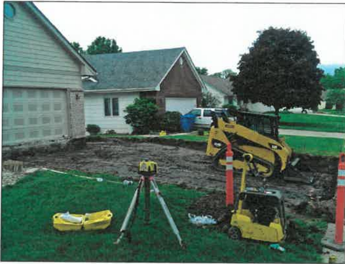
Step 1 Removal of concrete and excavation
