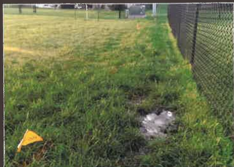
Lack of water infiltration
