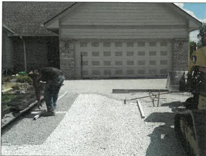
Step 3 Leveling and compacting aggregate
