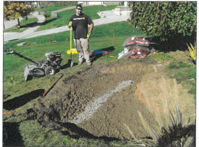
Step 2 Excavate existing soil
