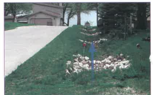
Dickinson County Bioswale
